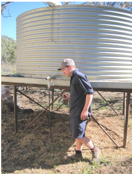
Reece inspecting the water tank
